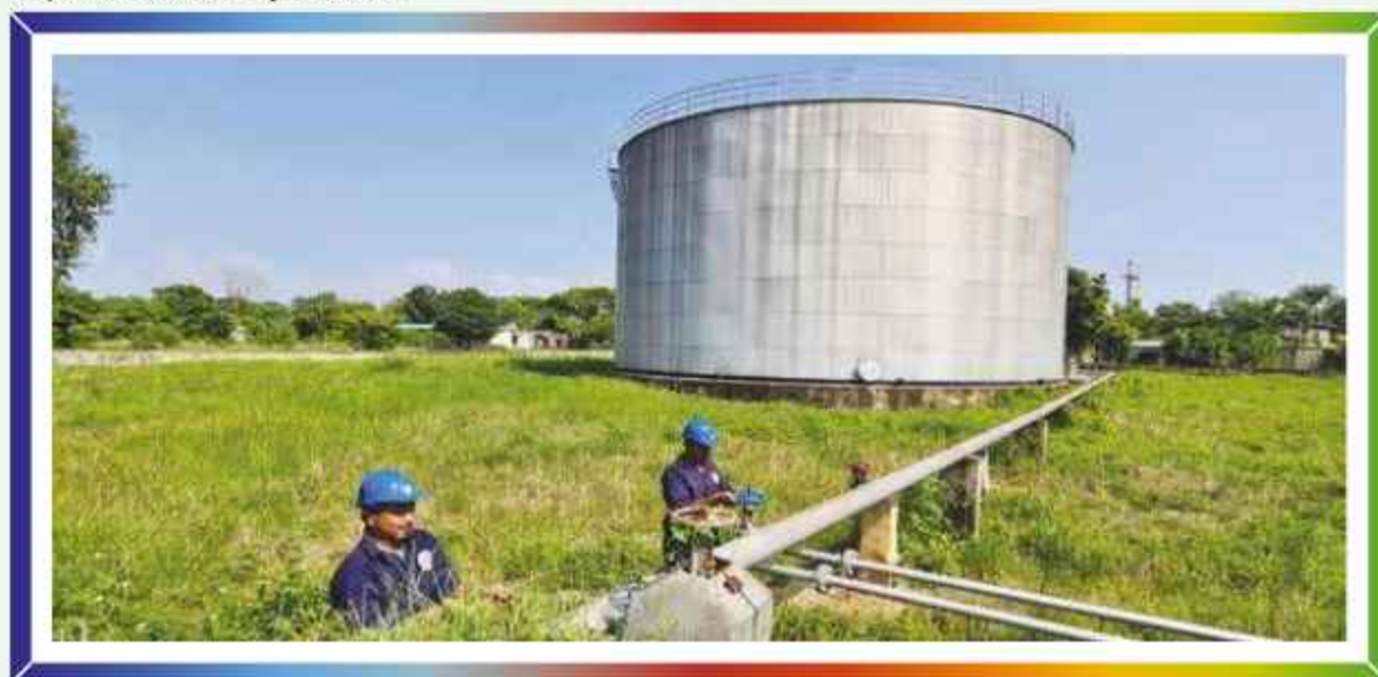
Preparation for delivery of Condensate stored in tanks at Ashugarj.
